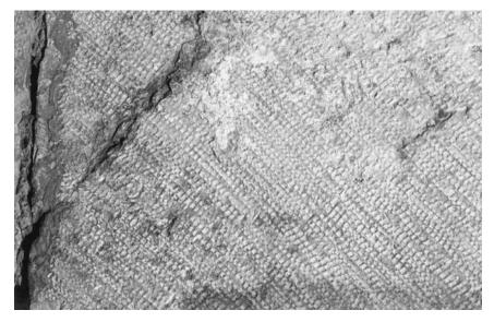
Figure 71 Masonry (diagonal tooling) (photograph by the author).
